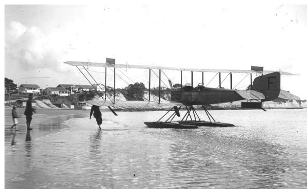
Figure 9. The B & W Seaplane. Naval Constructor George Westervelt designed this seaplane for a lumber-man who had become interested in aviation. William Boeing built two of these aircraft, and then a few more later on.
