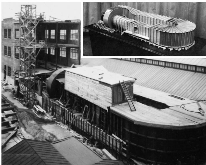
Figure 9. Wind Tunnel under construction (c1913) for the Navy’s Aerodynamics Laboratory, Washington Navy Yard (inset shows replica model).
