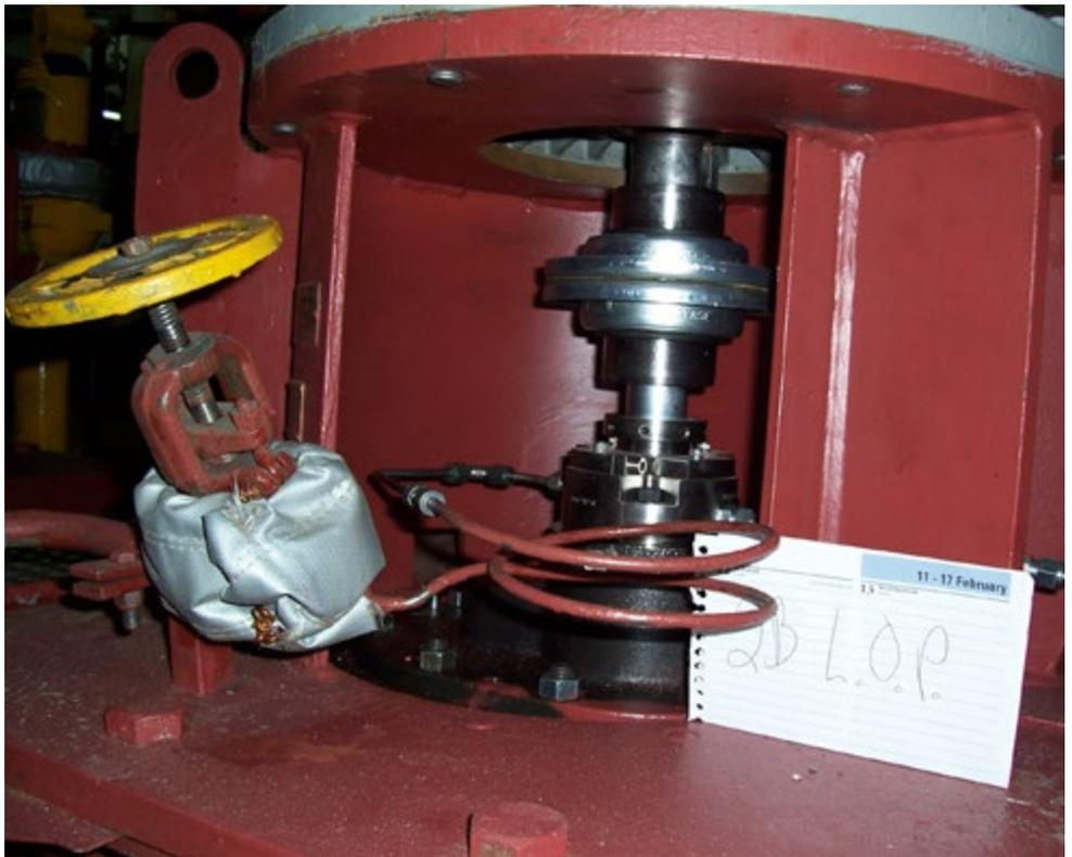
Lube oil service pump after installation of the dry flexible coupling. (U.S. Navy photo by Brett Franks/Released)
