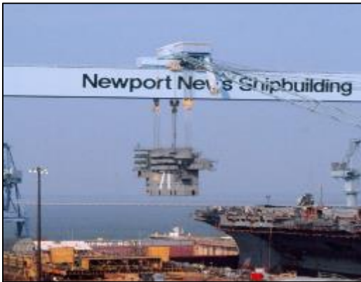
1970 -1990's – First Nuclear / First Modular Construction 10 Carriers / ~1090 Ft / 85K Tons
