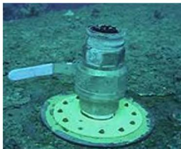
Figure 5-7. Valve Threaded onto Flange
