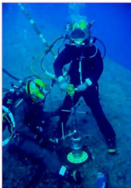
Figure 5-8. Two Divers Operating a Hot Tap Device
