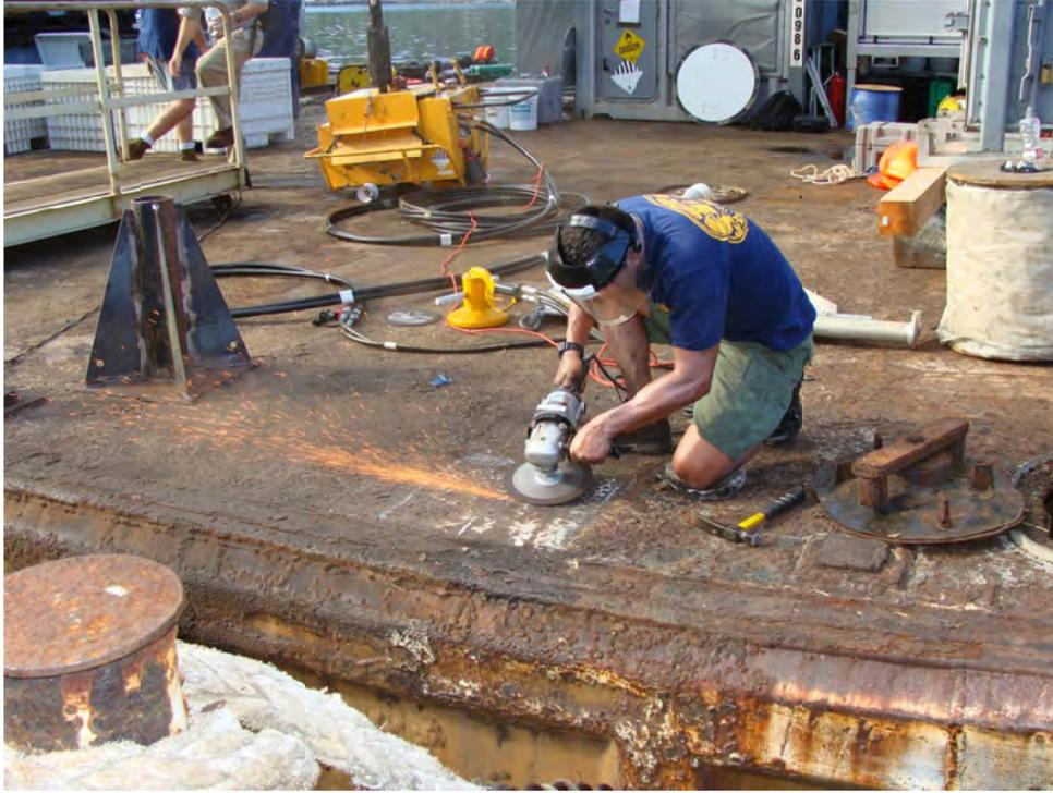
Figure 5. Diver Preparing Barge Deck for Davit Installation
