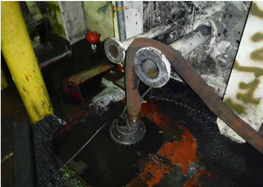
Figure 3-7. Pump rigged in sump of Cargo Hold 3A. Evidence of oily residue on bulkhead bears witness to higher water levels.
