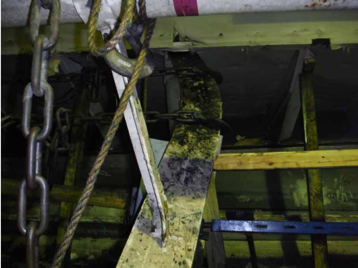
Figure 8: Frame 45 Damaged & Shored
