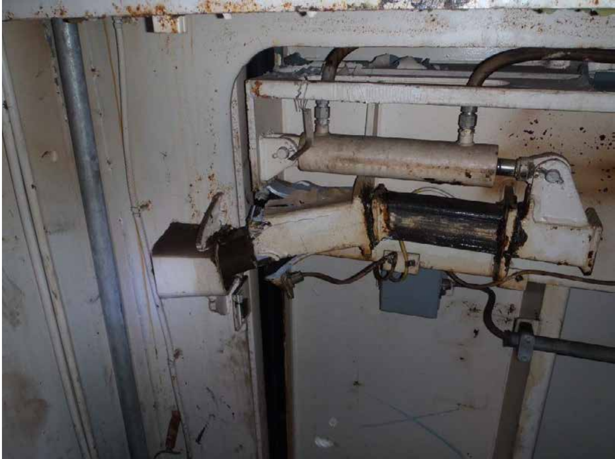
Figure 9: Dislodged Watertight Door
