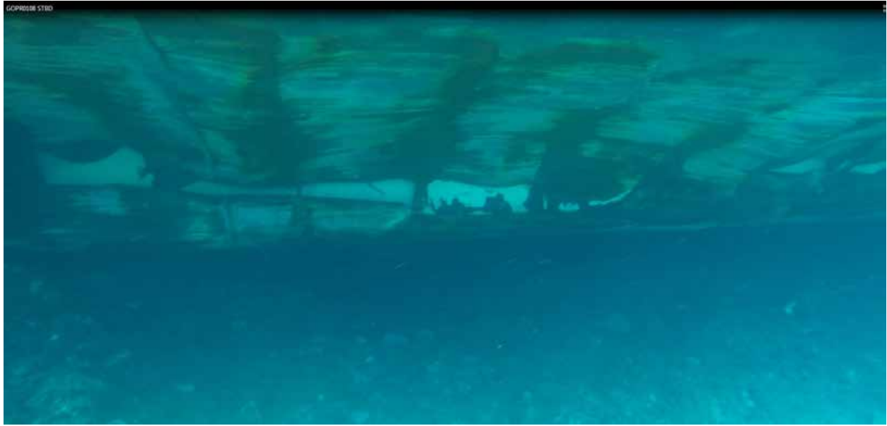
Figure 7: Hull Damage (Stbd)
