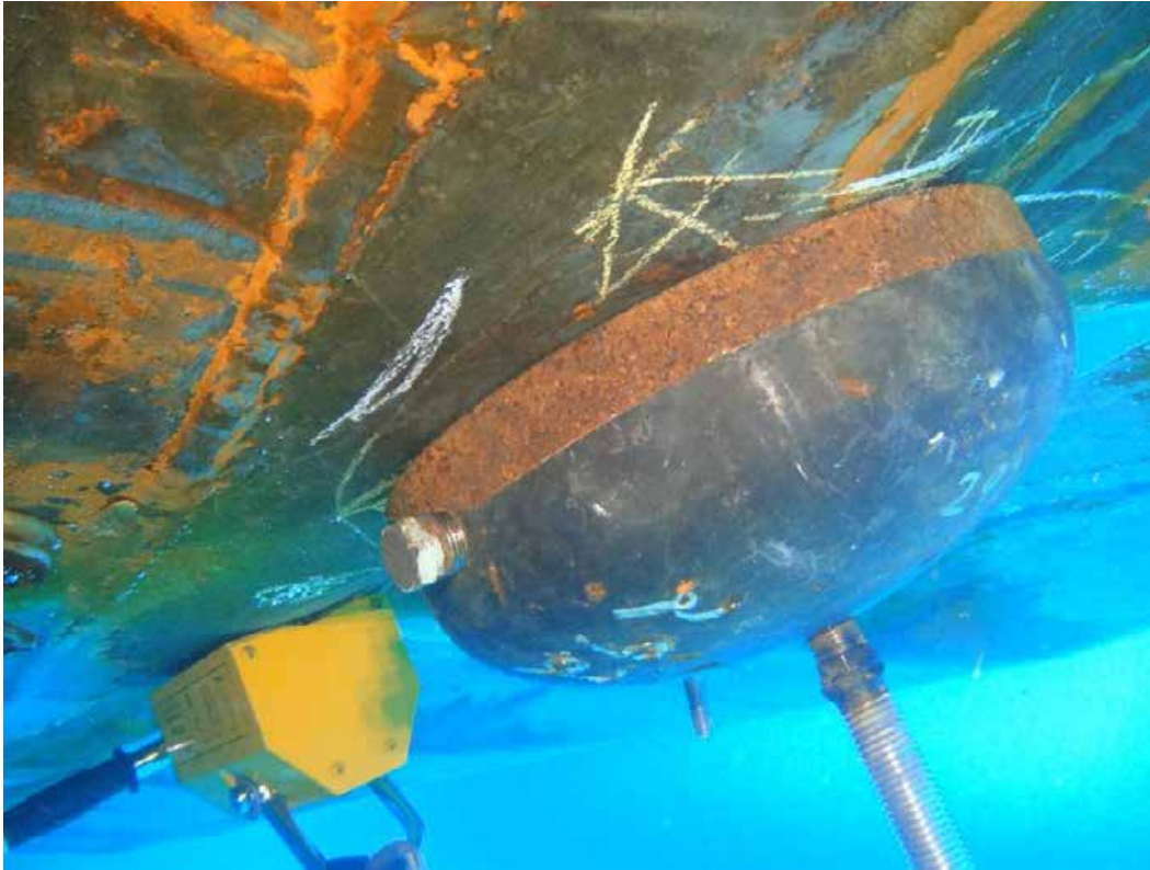
Figure 4-4. Dome patch templating on port side of USNS KOCAK. The repair team used dome patches to compensate for the distortions the hull plating.
