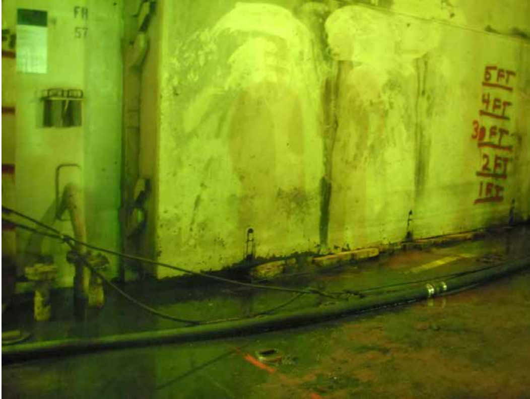
Figure 3-3. A view from Hold 4 looking aft at the water tight door.
