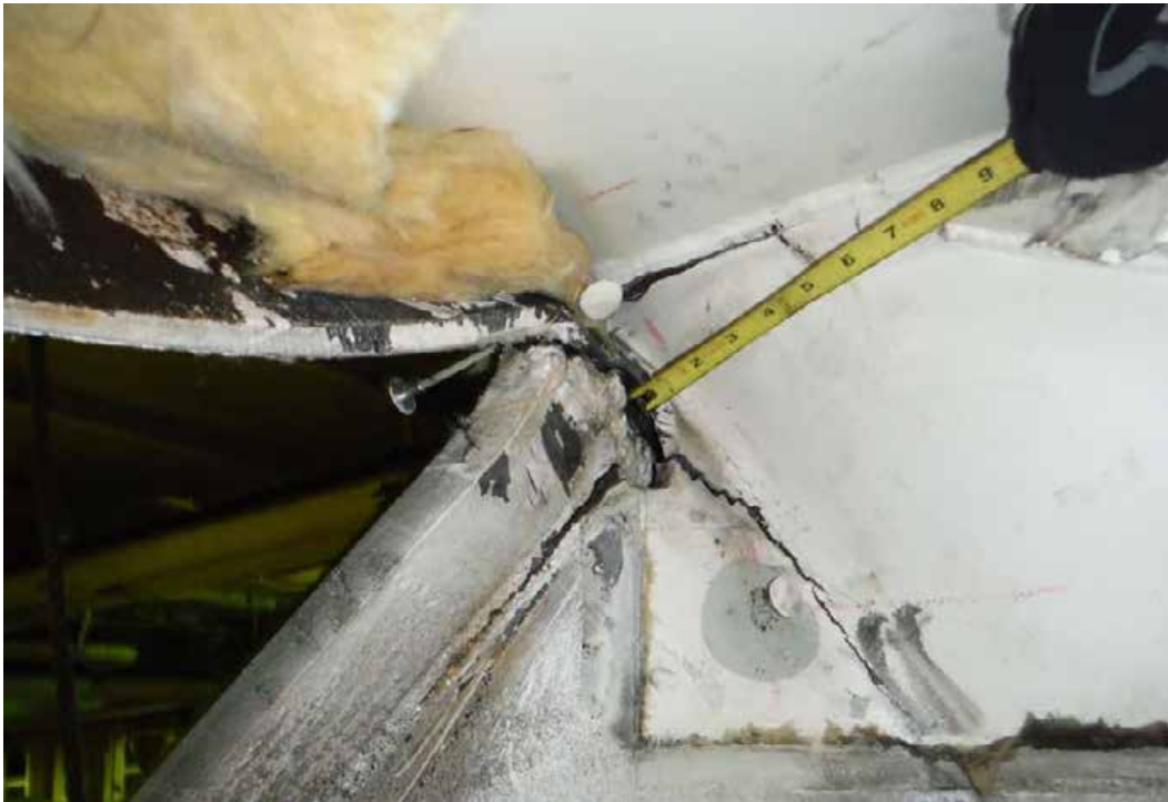
Figure 3-8. Bulkhead Stiffener Cracks in Hold 3A.
