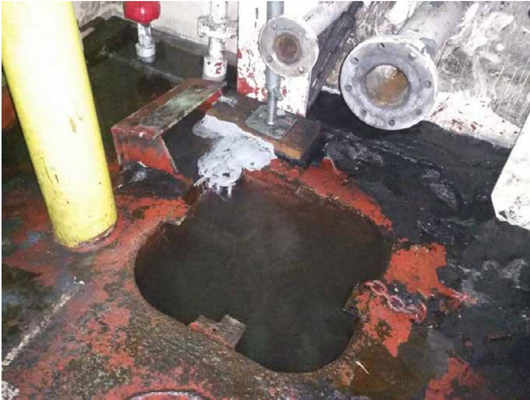
Figure 3-12. Patched and cleaned Hold 3A sump awaiting float off.
