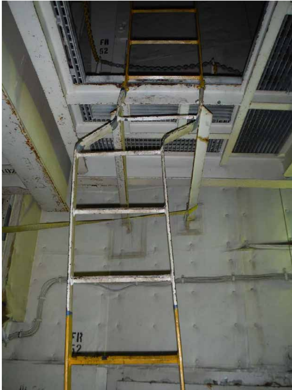
Figure 3-10. Hold 4 port side tank top buckling resulted in stress on this ladder.
