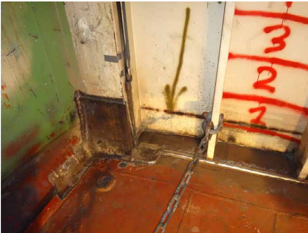
Figure 4-6. 4-4A Watertight door repairs. Left hand corner welds were strengthening and sealing outboard bulkhead of compartment and adjacent wing fuel tank.
