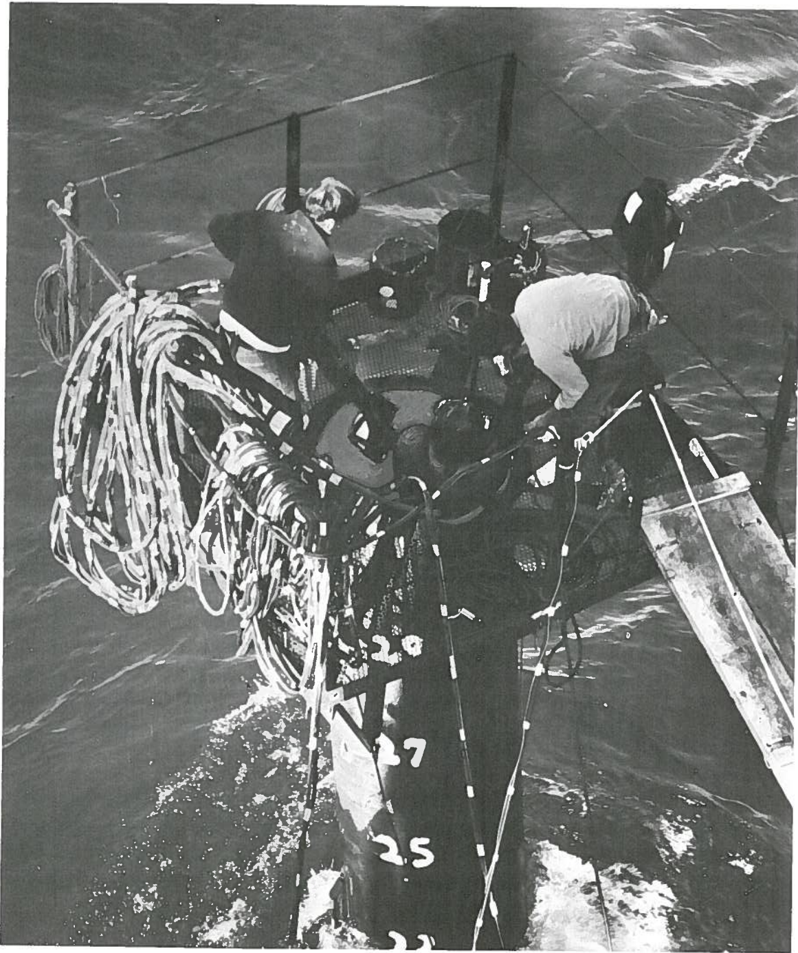
Diver is assisted by tenders as he descends through cofferdam to foam compartments of submerged bow section.
