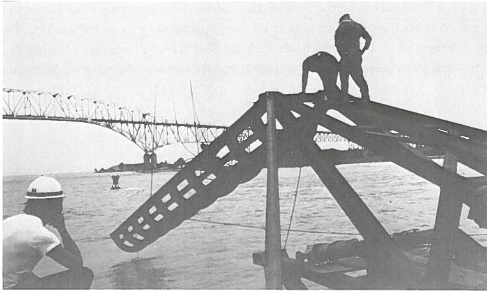
Cofferdam guide, 28' long, cradles cofferdam during lowering into place against sunken bow section. A-frame keeps guide and cofferdam clear of barge. Screw-type jack controls guide angle.
