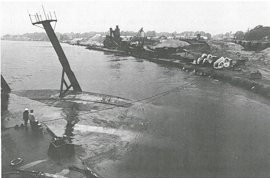
Bow broke surface 100 feet from shore near end of all night pull, 21-22 September, after 3½ months on river bottom.
