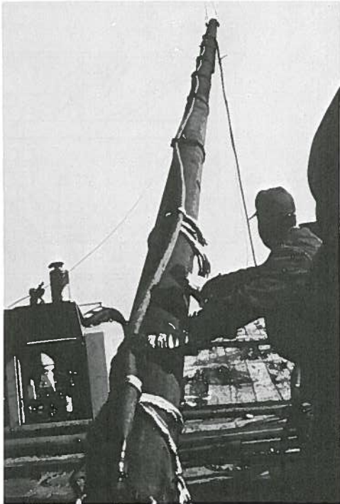
Air compressor feeds compressed air through air hose down to base of airlift pipe (left). Presence of air in water column inside airlift pipe creates pressure differential, forcing water, with coal nuggets and sediment, up through pipe for discharge into river (right).
