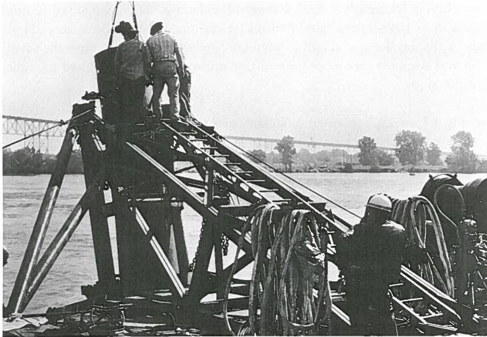
Cofferdam didn't seat properly against bow bottom. Screw-type jack carried away and both cofferdam and A-frame were damaged. Salvors here are extricating cofferdam following the failure.
