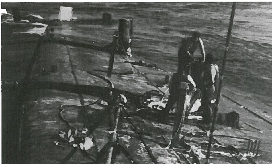
Salvors tend diver foaming cargo hold from access tube. Fittings are also in place for foaming from topside by probe method. Chains are rigged to pull points on port side.
