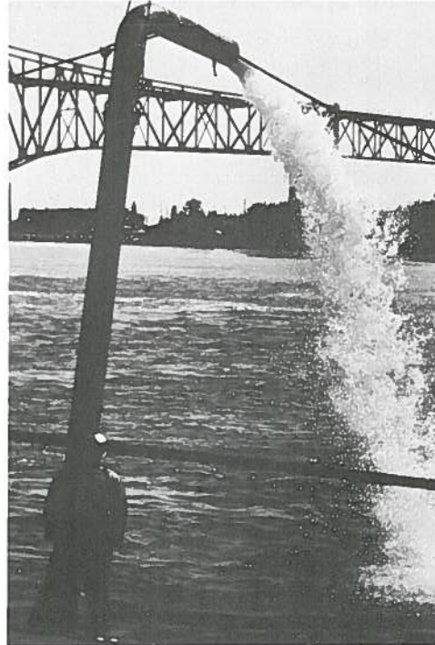
Air compressor feeds compressed air through air hose down to base of airlift pipe (left). Presence of air in water column inside airlift pipe creates pressure differential, forcing water, with coal nuggets and sediment, up through pipe for discharge into river (right).
