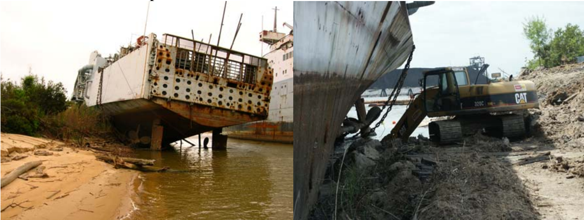
Figure 14. Ex-SHADWELL hard aground and at the beginning of land based excavation.
