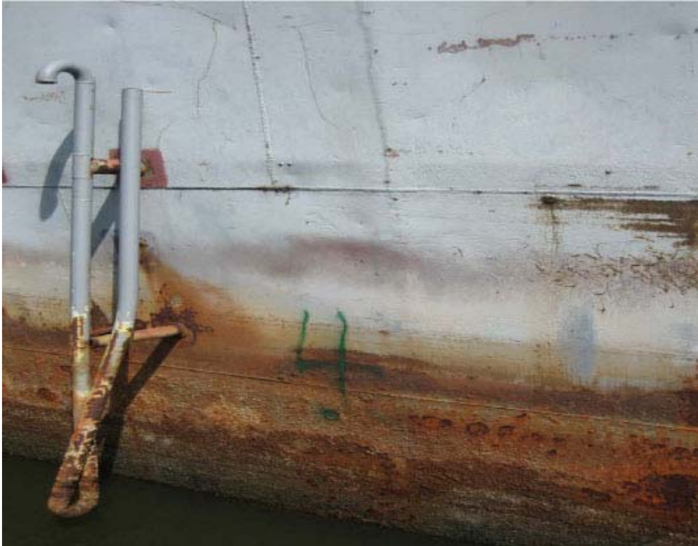
Figure 11. Location 4, Frame 64. Readings were taken both above and below the weld seam to the right of the location number. Note hollowed shell plating between frames
