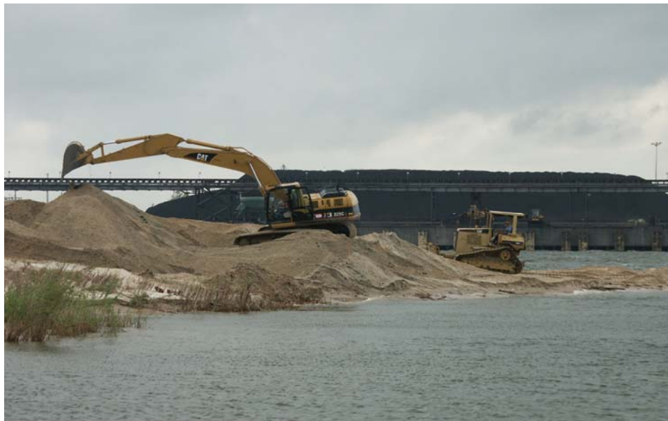
Figure 10. South West corner of the cove on Little Sand Island. Machinery moving sand removed from Ex-SHADWELL's planned moor.
