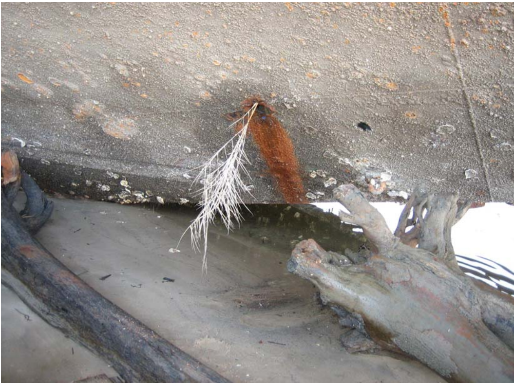
PHOTO - 3 - DISINTEGRATED WELD IN SEAM - FR 100 PORT
