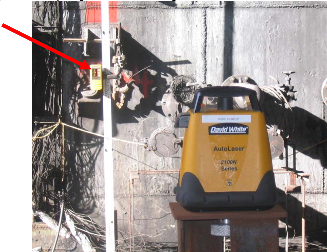
Figure 11. Davis White rotating laser level (to the right) and receiver/measurement point to the left (highlighted by arrow) in well deck of Ex-SHADWELL
