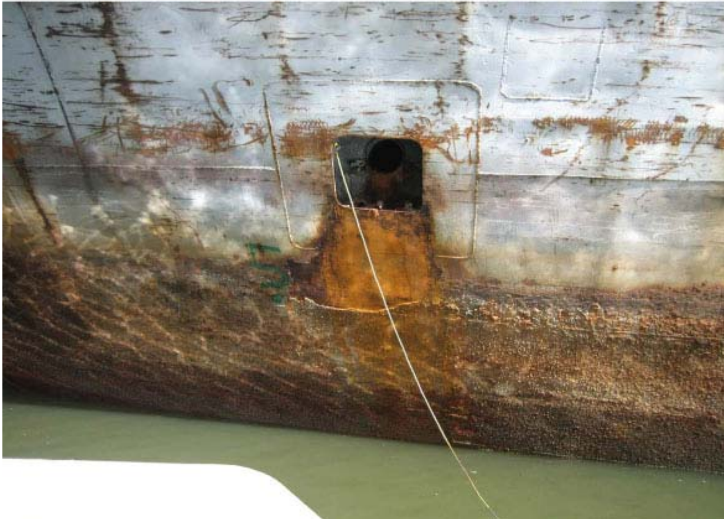
Figure 12. Location 5, Frame 79. In way of seachest for clean ballast.
