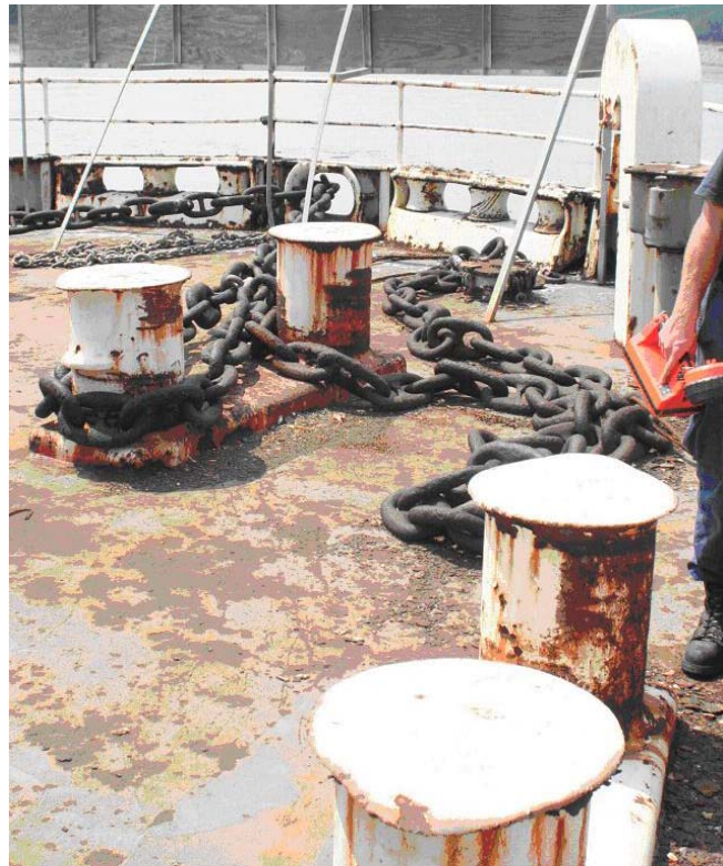
Figure 14: ex-STATE OF MAINE Port Aft Bits
