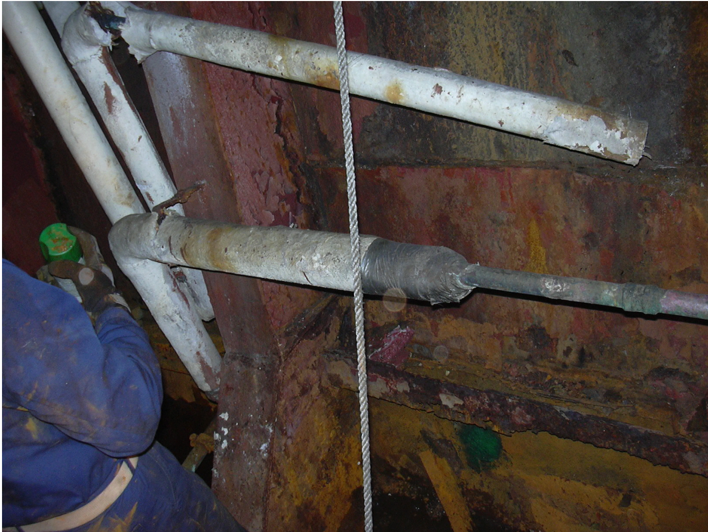
Figure 5. L-8 wasted in stbd. engine room.
