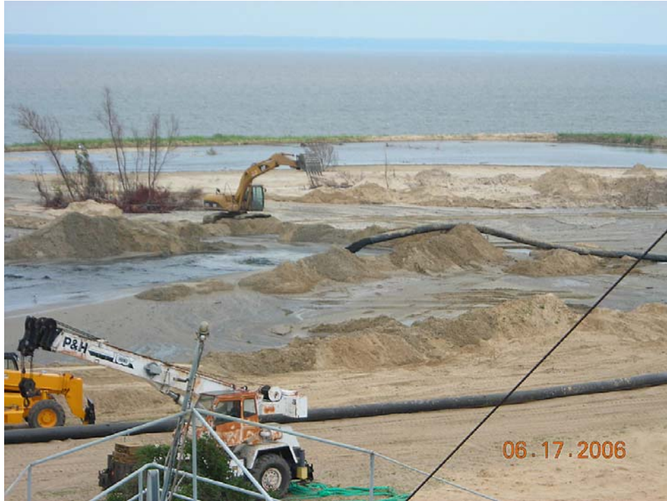
Figure 9 Little Sand Island spoil site. Earth moving equipment arranging sand during a dredging break.
