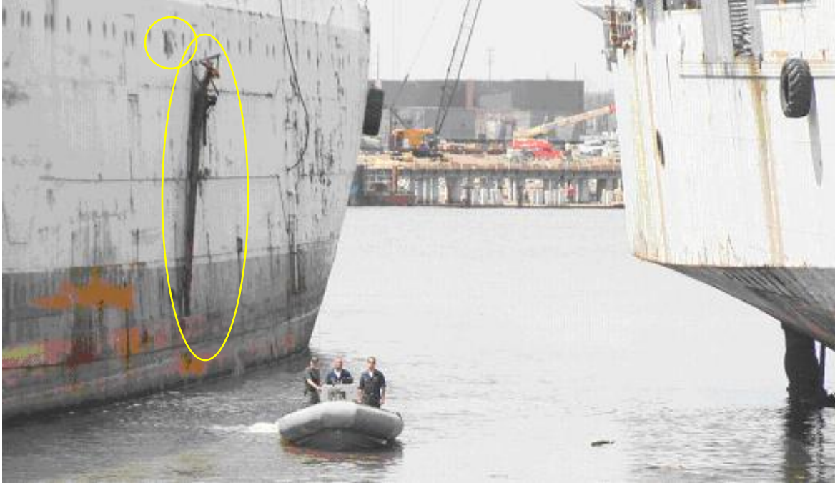
Figure 3: Structural damage to ex-STATE OF MAINE
