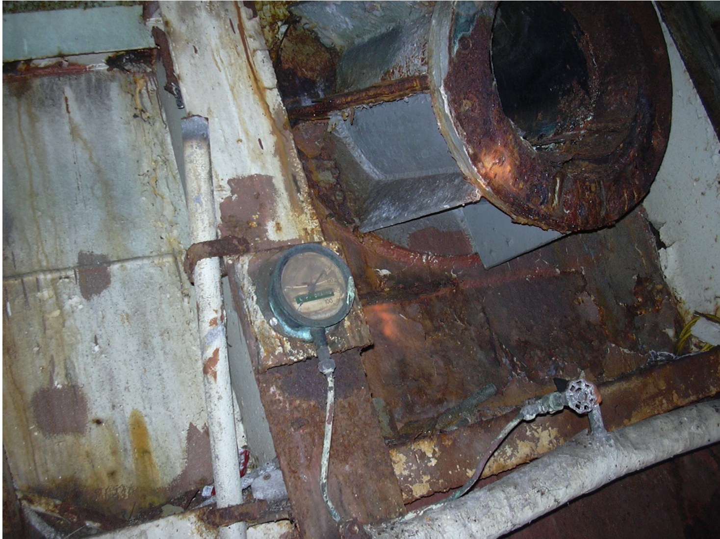
Figure 6. Wasted 6X4 longitudinal above turn of bilge in stbd. engine room.
