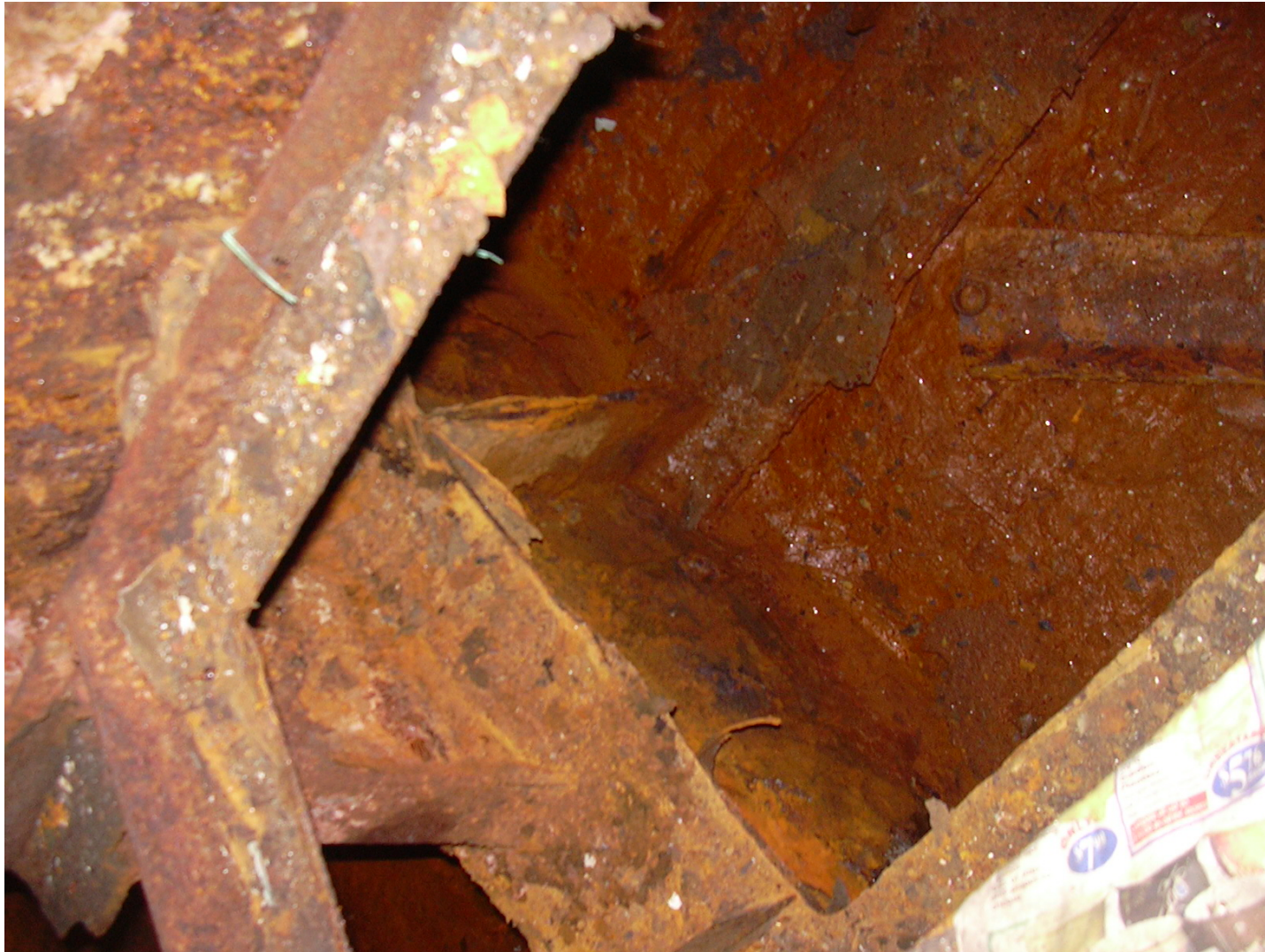
Figure 2. Transverse beam intersecting longitudinal L-7 in port engine room.
