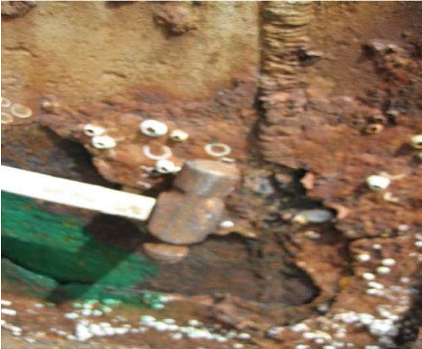
Figure 8. Area showing green location mark at Location 1, and area of chipped off scale.
