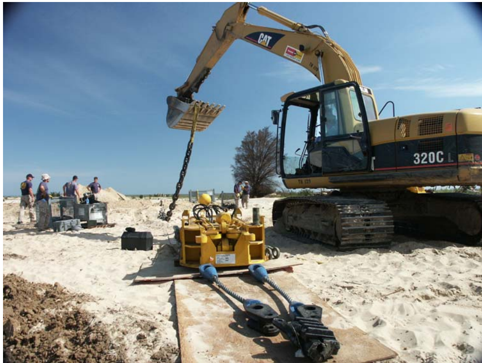
Figure 12. Excavator assisting MDSU ONE team in setting the anchor in a deadman. In foreground is the bridle assembly and 50-ton hydraulic cable puller and to the left is the control panel and new electronic tension measuring device.
