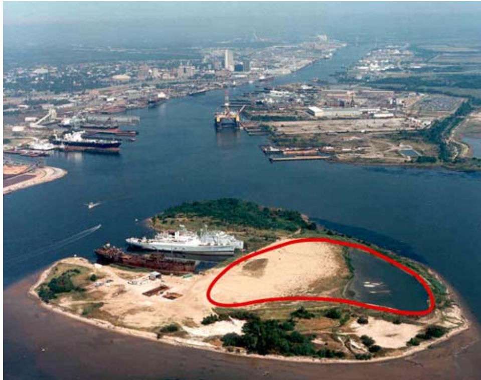
Figure 4. Little Sand Island. Cove containing Ex-SO MAINE and Ex-SHADWELL to the left. Dredge spoil area and berm location drawn in red to right. This picture was taken well before Hurricane Katrina and the third vessel shown in the image to starboard of Ex-SO MAINE was not present at the time of the storm.
