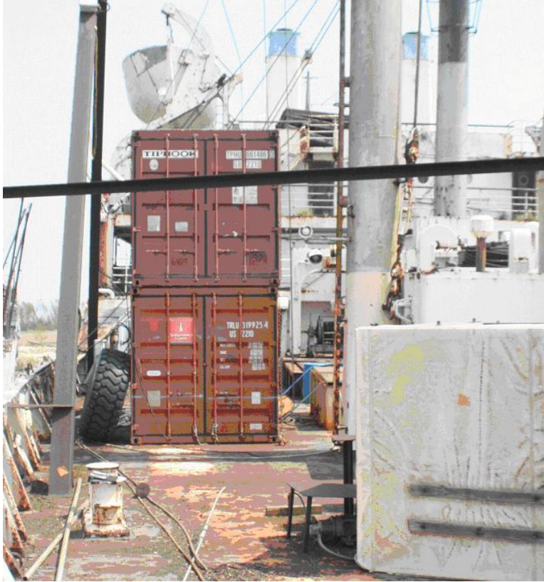
Figure 9: ex-STATE OF MAINE Port Main Deck
