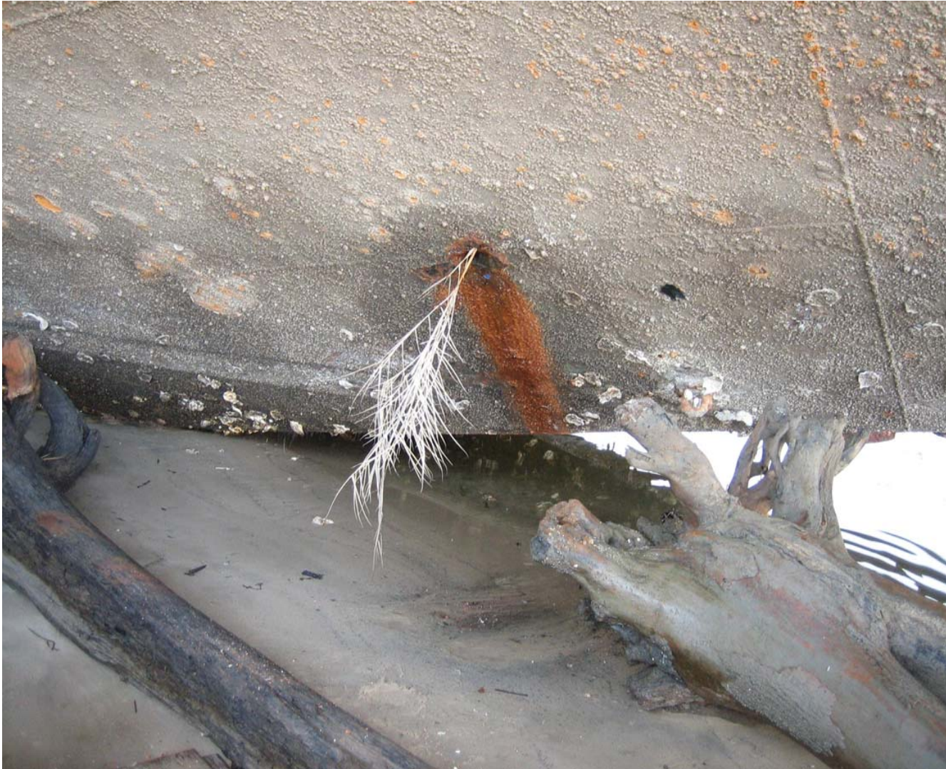
Figure 16. Disintegrated weld in seam near FR 100 port.
