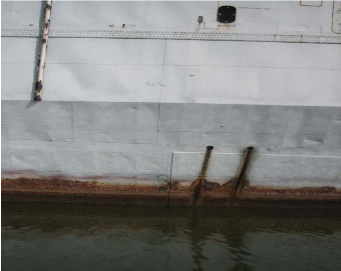
Figure 9. Location 2, Frame 36. Readings were taken aft of the doubler plate in areas both above and below the scale line.
