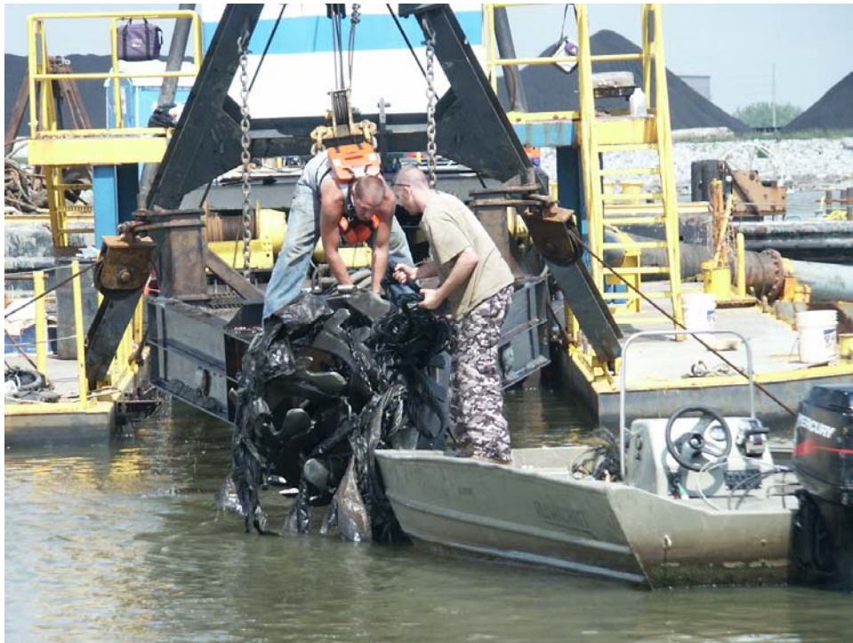
Figure 7. MDSU and dredge operators work to clear large dredge cutter head of debris encountered during dredging operations
