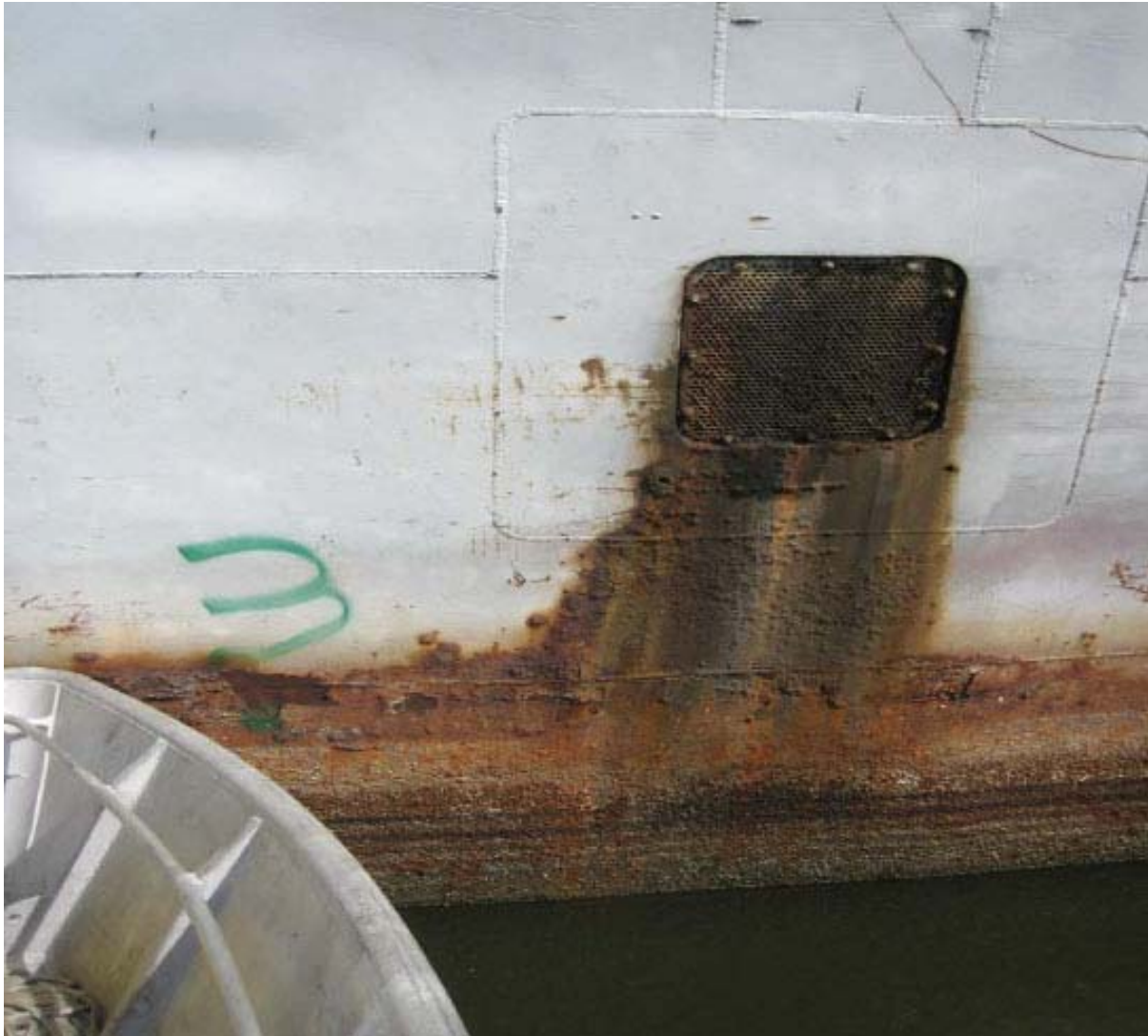
Figure 10. Location 3, Frame 49 in way of seachest for clean ballast.
