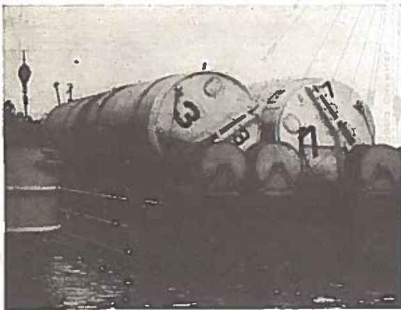
FIGURE 3.—Salvage pontoons were towed to scene on barges.
