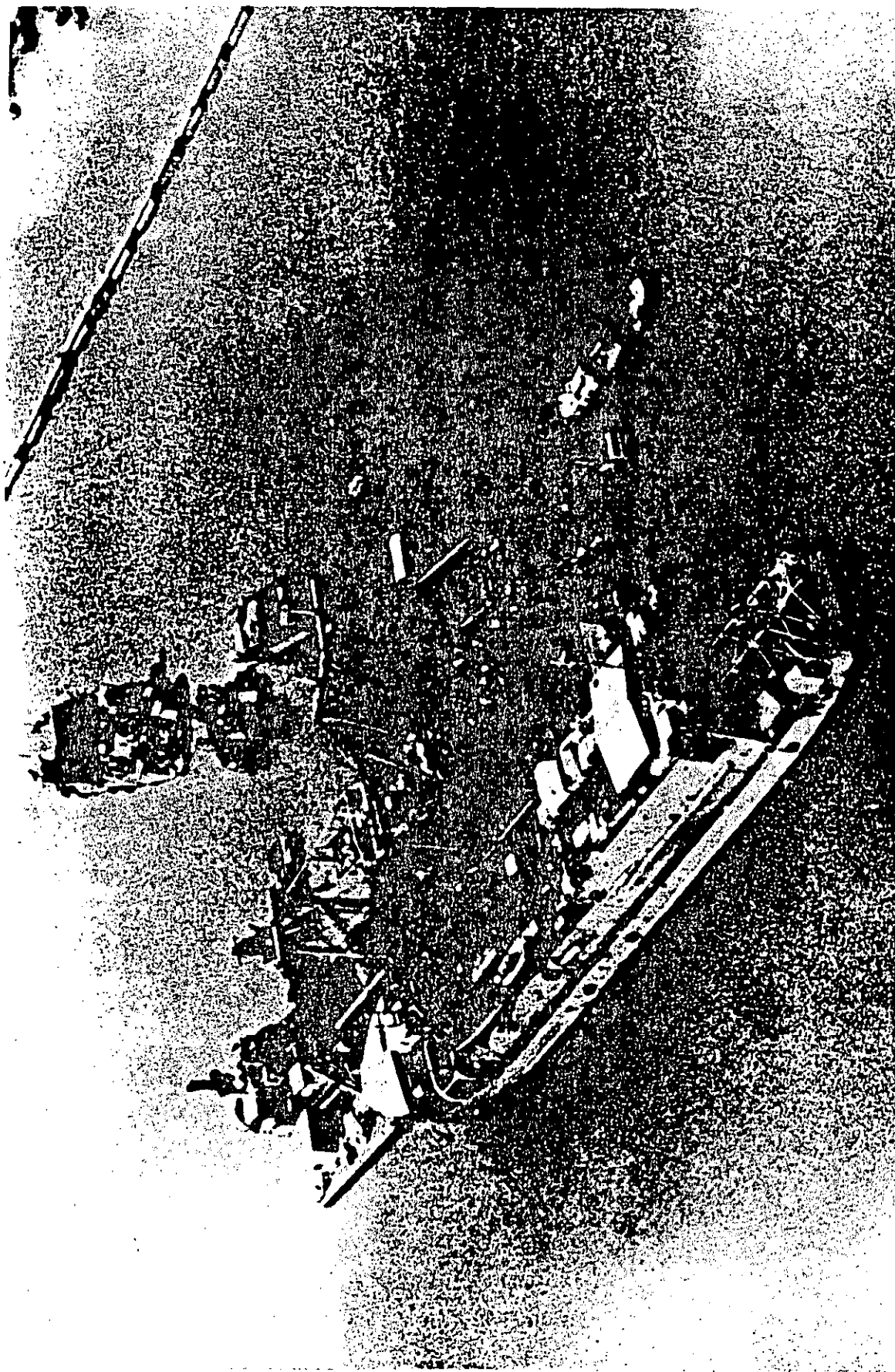
AERIAL VIEW OF THE JAMAICA BAY SALVAGE OPERATION. FIG. 14 NO. 3
