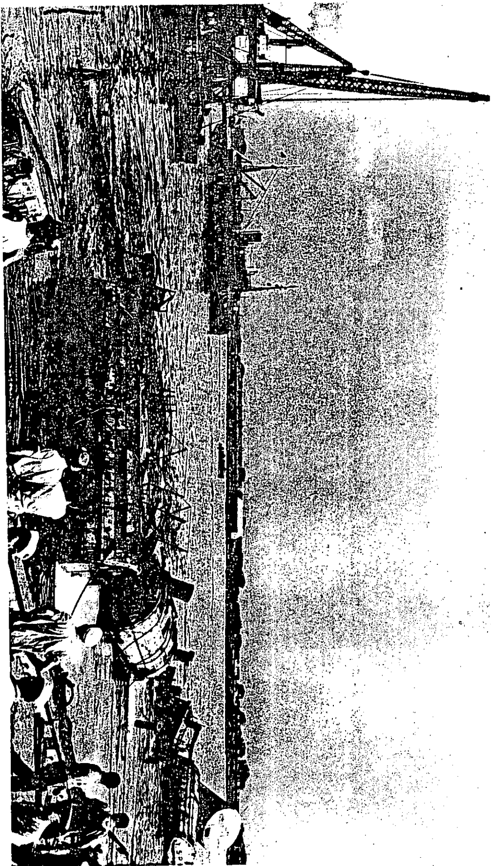
WITH THE ASSISTANCE OF SUBMARINE SALVAGE PONTOONS, THE USS OGLALA IS RIGHTED ON 23 APRIL 1942. FIG. 12 NO. 5
