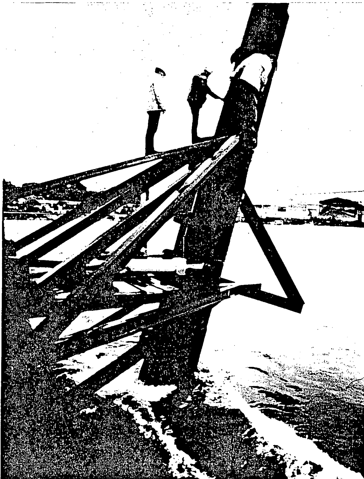
LOCATING MECHANISM POSITIONING DIVERS ACCESS COFFERDAM. FIG. 15.11 NO. 2
