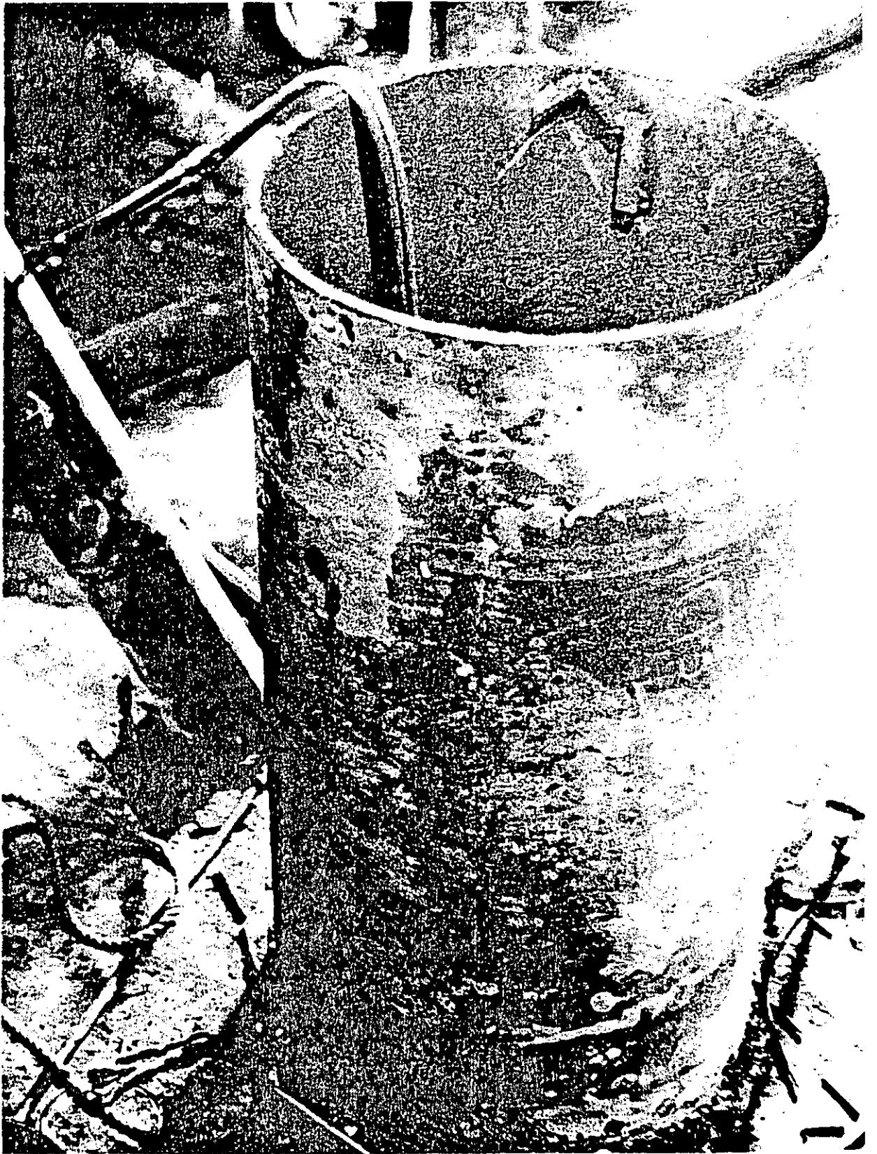
TWENTY-FOUR INCH COFFERDAM, PORT SIDE ON THE NEW JERSEY. FIG. 14 NO. 23
