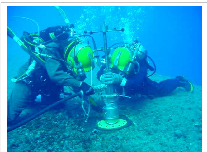
Figure 6-4. U.S. Navy Divers Installing Hot Tap System on Hull of Submerged Vessel.
