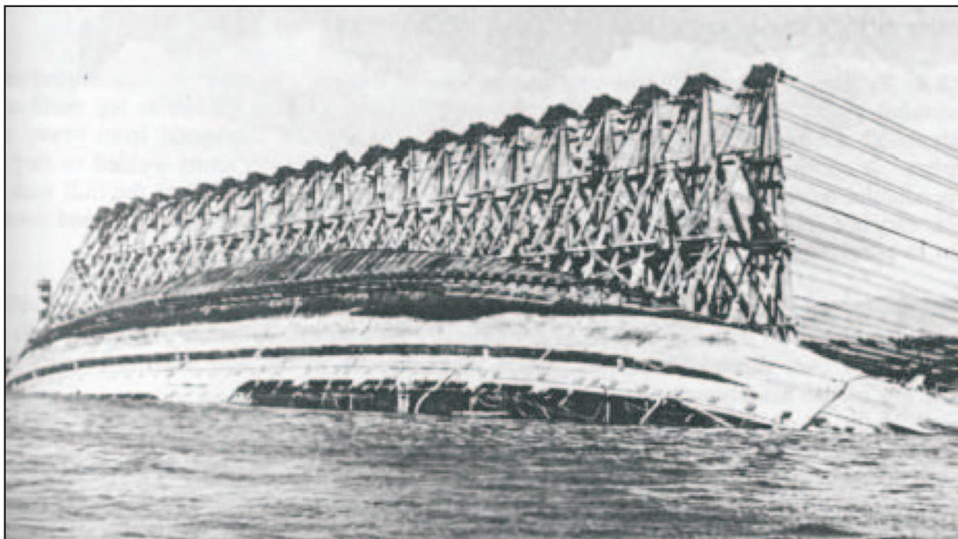
Figure 7-15. Braced-Girder Headframes on USS OKLAHOMA.
