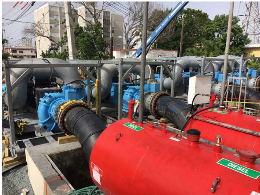
Malaria Pumping Site configured with temporary pumps.
