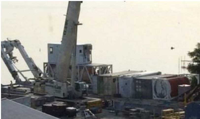
SAT FADS system installed on the barge in Seneca Lake, NY.
