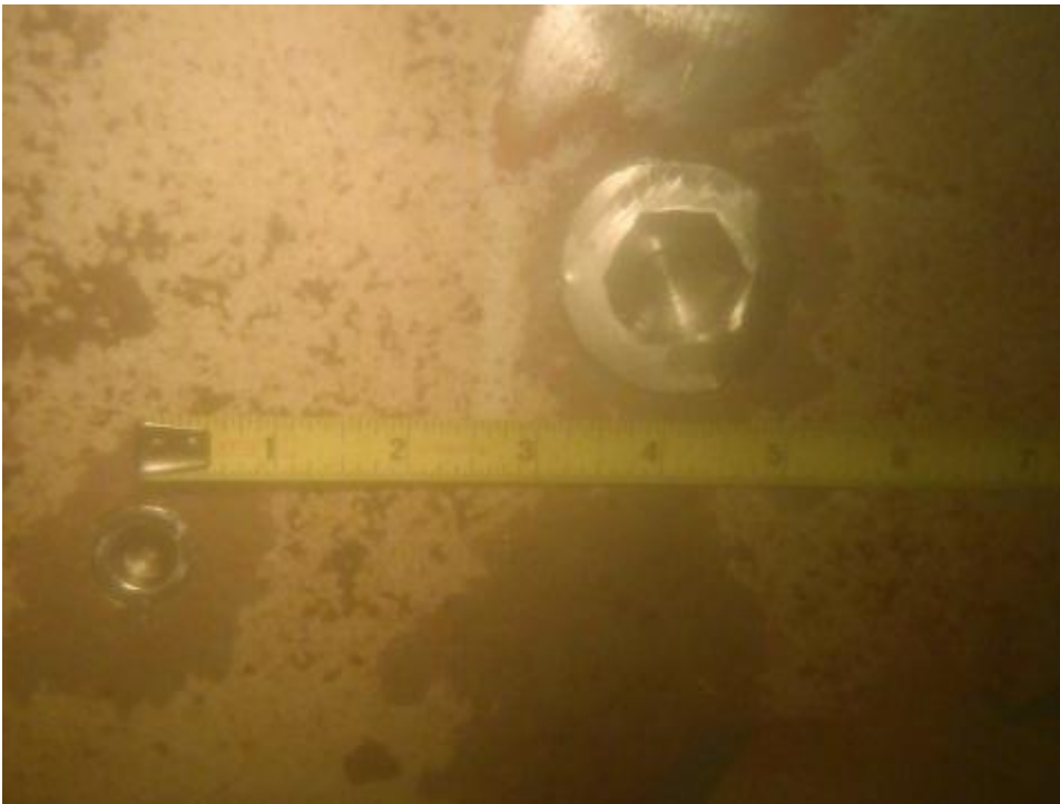
New plugs installed sealed the rudder retention access plate
