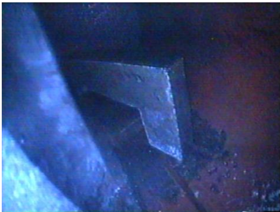
Stopper plate and lug plate were intact
