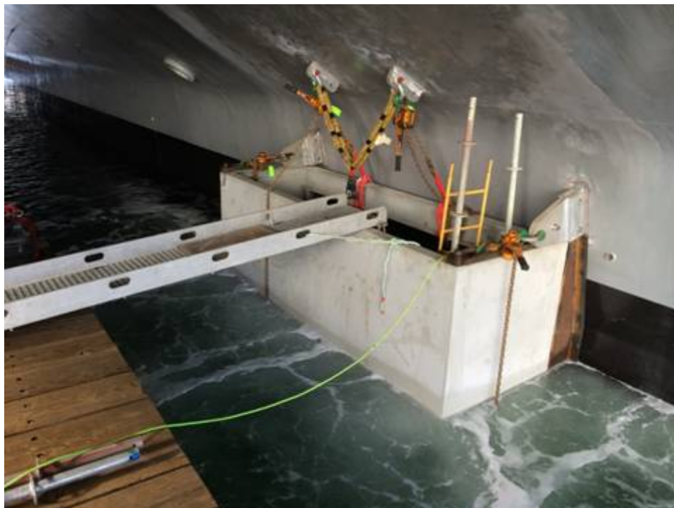
Cofferdam fastened securely to the ship and dewatered allowing repairs to skin valves to take place
