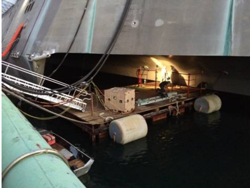
Welders installing a Hull Mounting Plate on the starboard side of the INDEPENDENCE hull.
