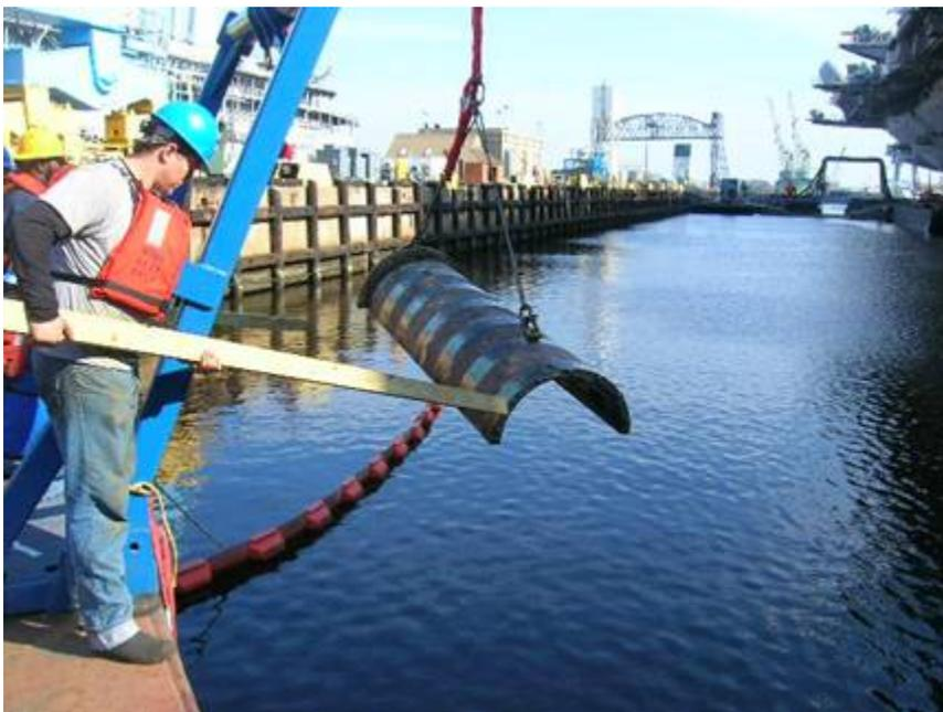
In this image, riggers can be seen guiding the newly re-staved bottom bearing half back over the barge to be hung from the A-frame and then installed on shaft number 4 (blue structure seen to the left of the bearing).
