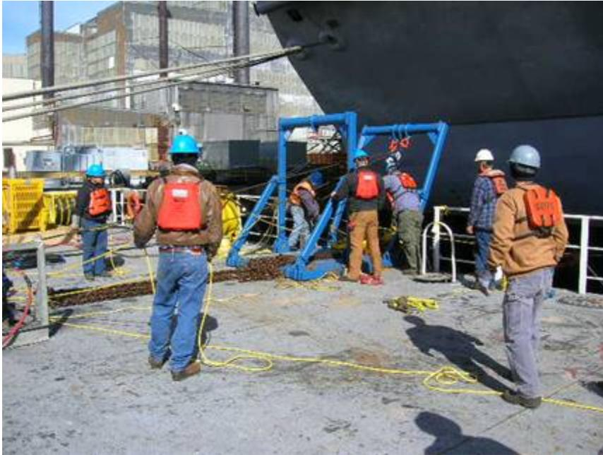
Tuggers were installed to aid the divers in handling heavy equipment in the water and under the ship. For example, 50-ton hydraulic chain hoists (weighing about 3,000 lbs) had to be rigged under the vessel for lifting the shaft and propeller (weighing about 100,000 lbs) enough to remove the lower half of each of the bearings.
