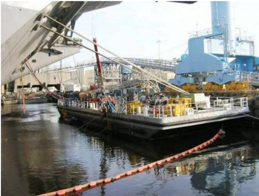
The first task was to rig work barges port and starboard off the stern of IKE to support the divers and rigging the heavy equipment and bearings from under the ship to the pier. Shown here is the starboard barge, used for rigging only. The port barge was set up the same for rigging but is also where the dive station was set up.
