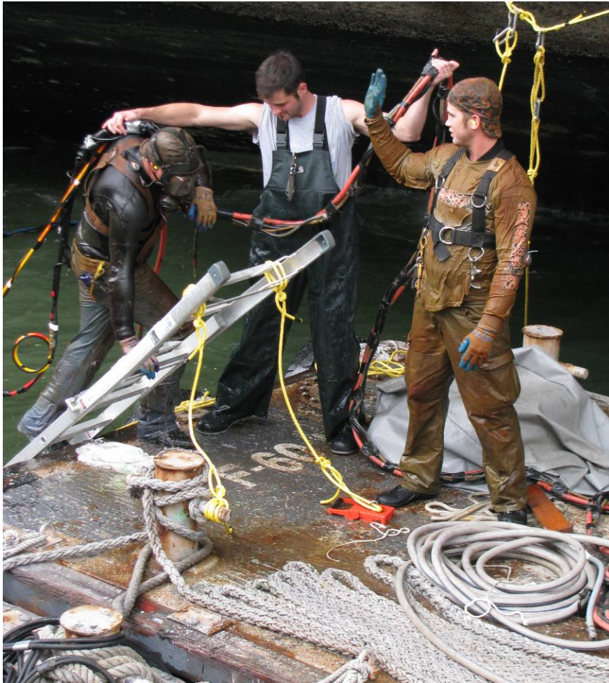
Phoenix divers returning to the surface in Sasebo, Japan after putting in a shift repairing USS DENVER's port shaft.
