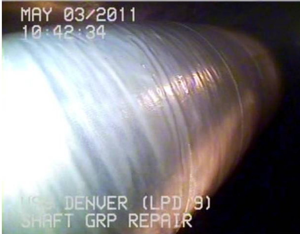
Completed repairs - shaft with new GRP covering before application of Hycote paint. This photo was taken from within the habitat.
