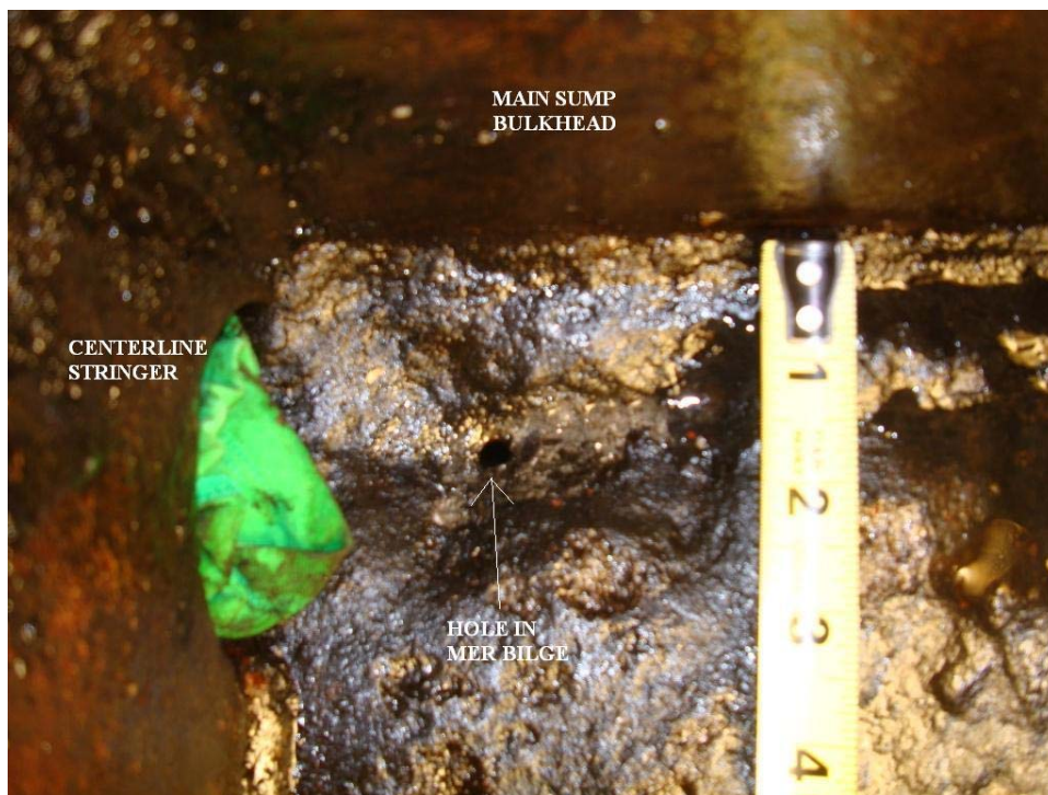
Close up image of the hole in the MER bilge.
