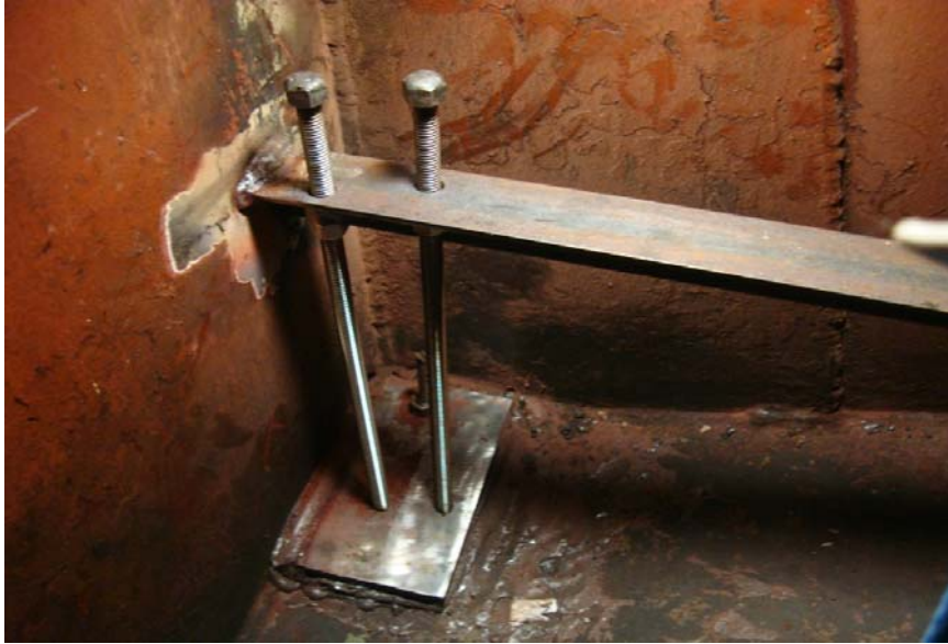
Metal patch stabilized by welded brace.
