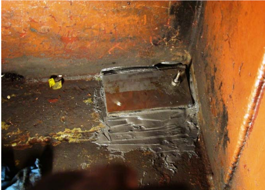
J-Hook and steel patch set in epoxy in bilge of MER.
