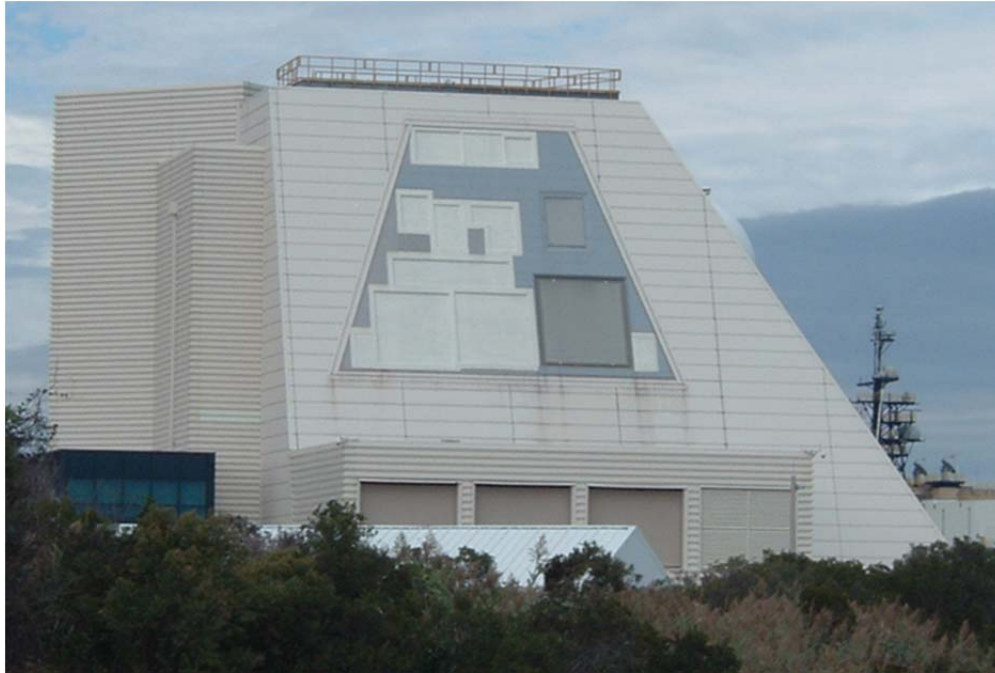
Exhibit 2-1: Existing South Elevation of Building V-003 with Carbon Composite Radar Array. The Two-Story Extension to the South Elevation is Visible Directly Below the Radar Array (Source: NAVFAC MIDLANT 2014a)
