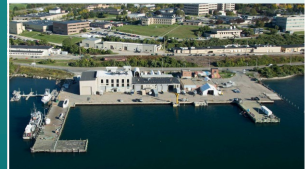
Narragansett Bay Test Facility, Newport, RI
