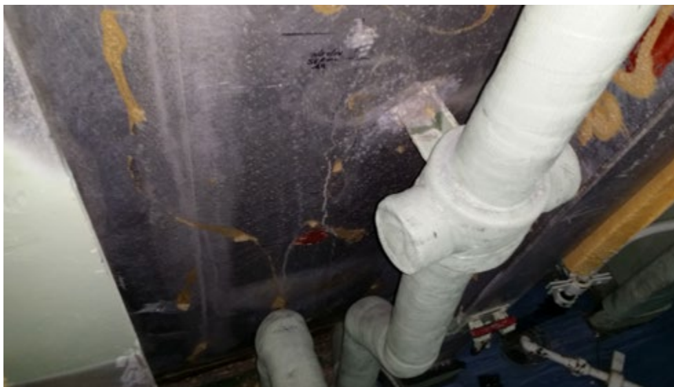
Before application of a composite patch aboard the USS Vicksburg (CG 69) in September 2014. (U.S. Navy photo by Bruce Wells/Released)
