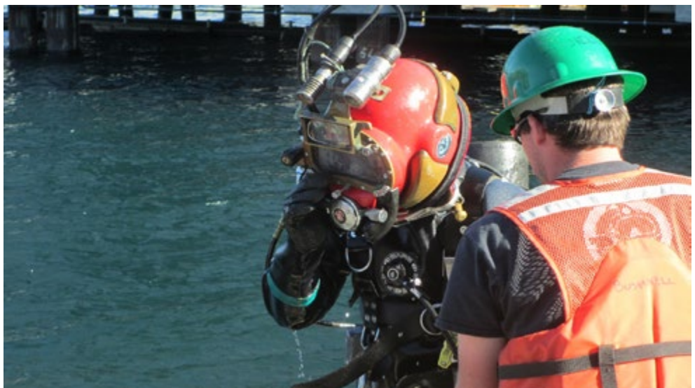
Top right: Pier 42, the primary support pier for Naval Surface Warfare Center, Carderock Division’s Acoustic Research Detachment in Bayview, Idaho in August 2014. The pier is showing its age, making it necessary to perform extensive repairs. (U.S. Navy photo by Alan Griffiths/Released)
