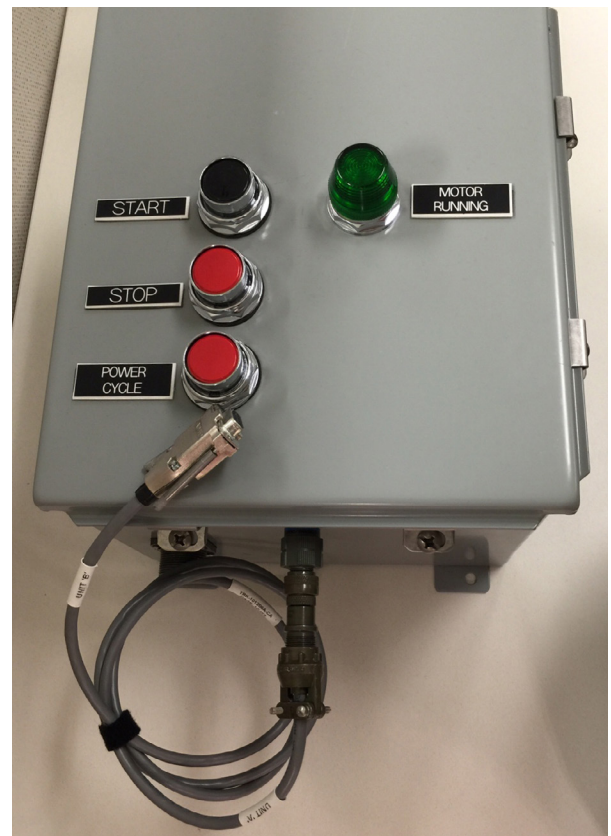
This photo shows the ventilation fan motor controller (VFMC) with the safety connector that Naval Ship Systems Engineering Station, Naval Surface Warfare Center Carderock Division mechanical engineer David Belch developed to reduce a Sailor’s exposure to 440 volts of alternating current when performing maintenance on the VFMC. (Official Navy photo by David Belch/Released)
