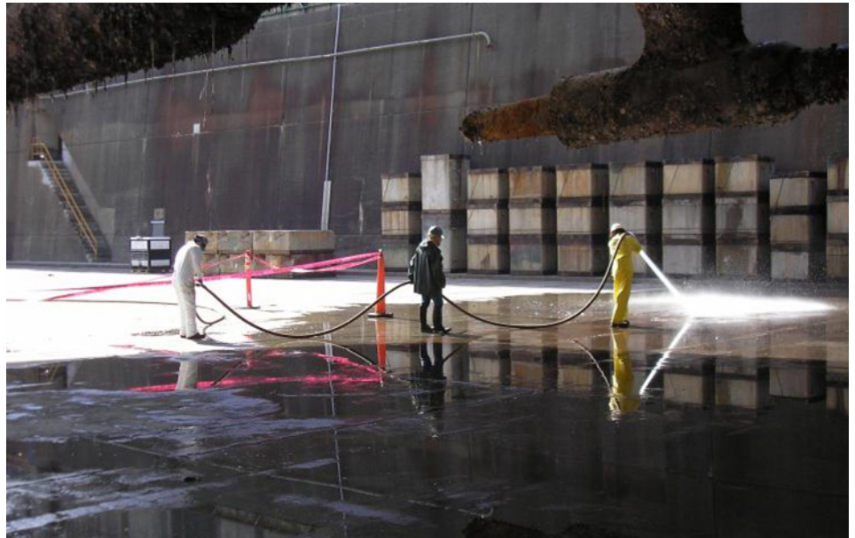
The current cleaning method includes a water wash-down performed using fire hoses, followed by shoveling or sweeping the accumulated sediment into 55-gallon storage barrels. This operation produces a large volume of contaminated water. The method is both time-consuming and heightens the potential for injury. (U.S. Navy photo/Released)
